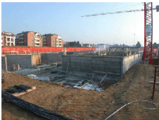
Fig. 5 - Piano interrato in c.a.
