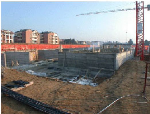
Fig. 5 - Piano interrato in c.a.
